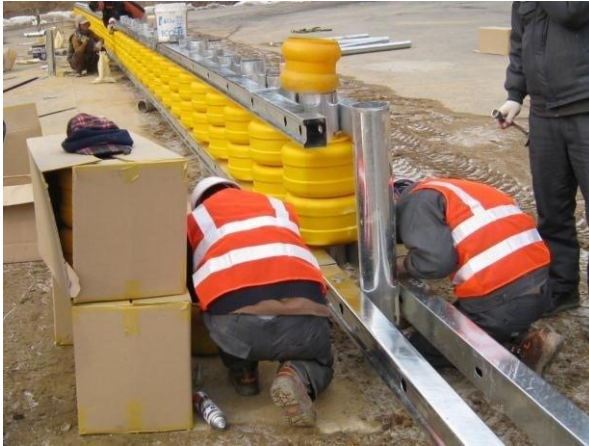
Figure 42: Checking poles and inserting barrier caps.
