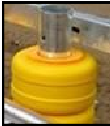
Figure 7: Image depicting the inner post of the safety roller barrier.
