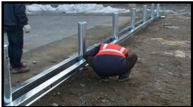
Figure 32: Assembly of the sleeve rail.
