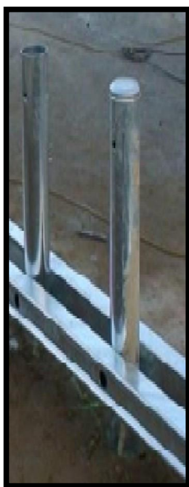
Figure 5: Supporting posts required for the safety roller barrier.
