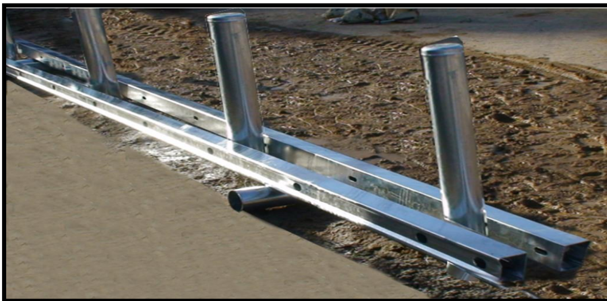
Figure 33: Finishing assembly of lower guardrail.
