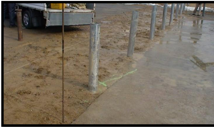
Figure 26: Alignment checking with a string line.
