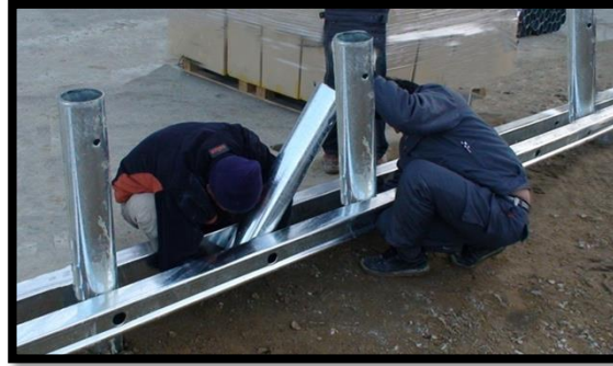
Figure 35: Assembly of intermediate post.
