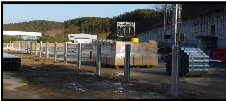
Figure 27: Finish with fixing the steel line posts.
