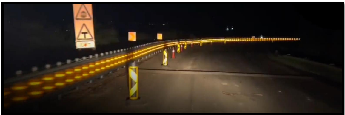
Figure 10: Guide reflectors to be used on safety roller barrier.
