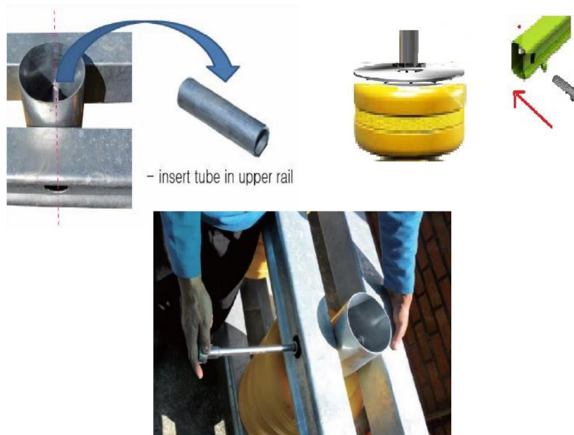
Figure 40: Placement of bolts.
