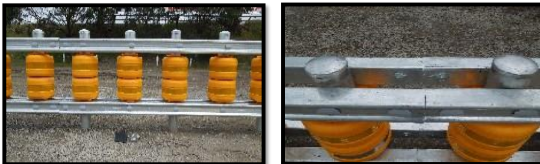
Figure 1: Image showing the safety barrier roller system.
