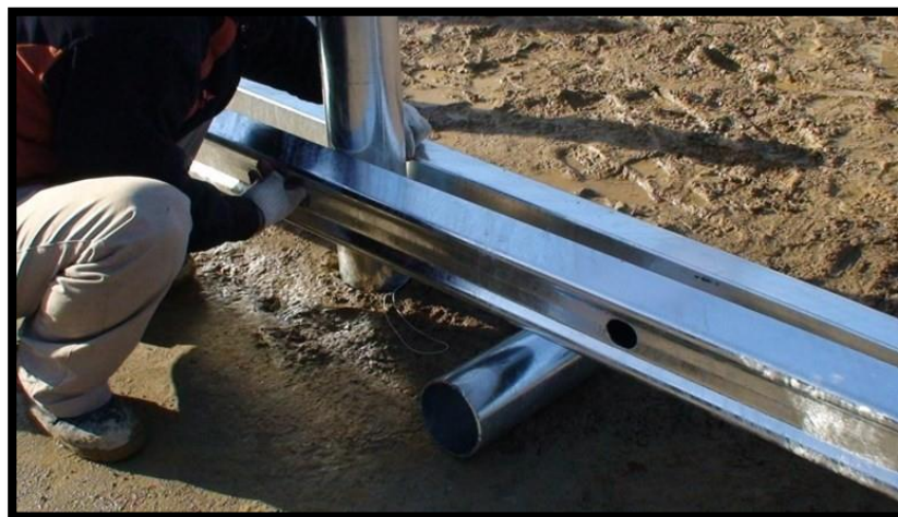
Figure 34: Gap indicated on the lower guardrail.
