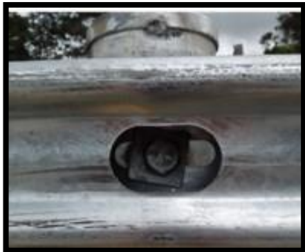
Figure 32: Assembly of the sleeve rail.
